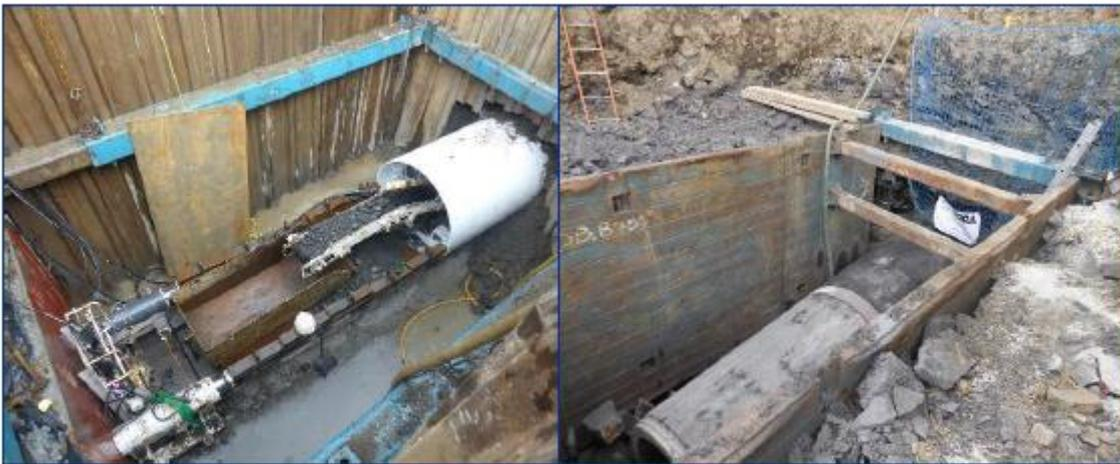
**Figure 16: Tunnel Jacking Launch Shaft**
